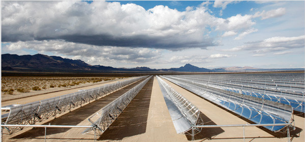
An Acciona solar thermal power plant, located south of Las Vegas.
