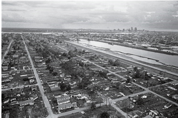
STILL DESOLATE: This section of New Orleans' Lower Ninth Ward is a mix of demolished houses and those still awaiting bulldozers.
