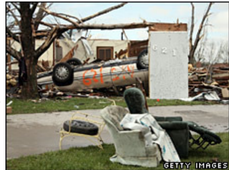
Greensburg suffered enormous damage after being hit by tornado last year.
